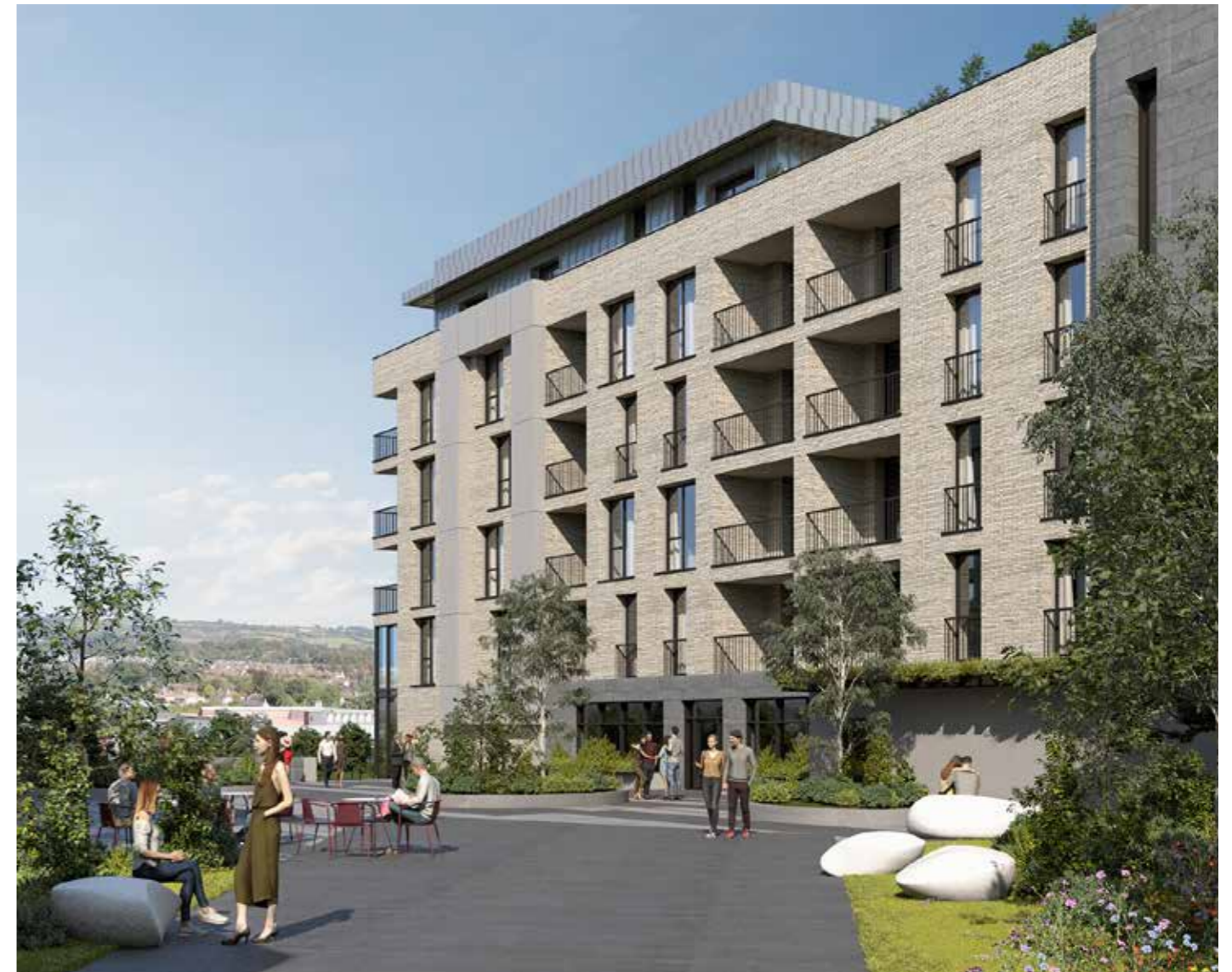
VIEW OF LANDSCAPED PODIUM
